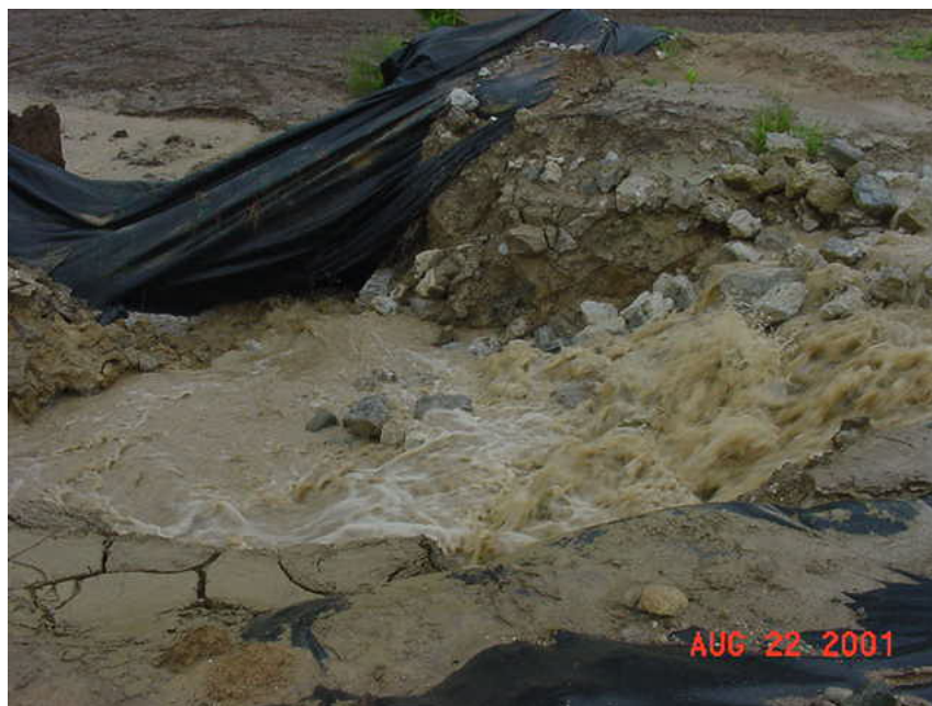
Photo 1: Improperly installed silt fence
