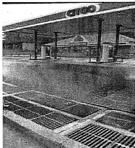
FIGURE 5-46 Delaware sand filter. SOURCE: Tom Schueler.
