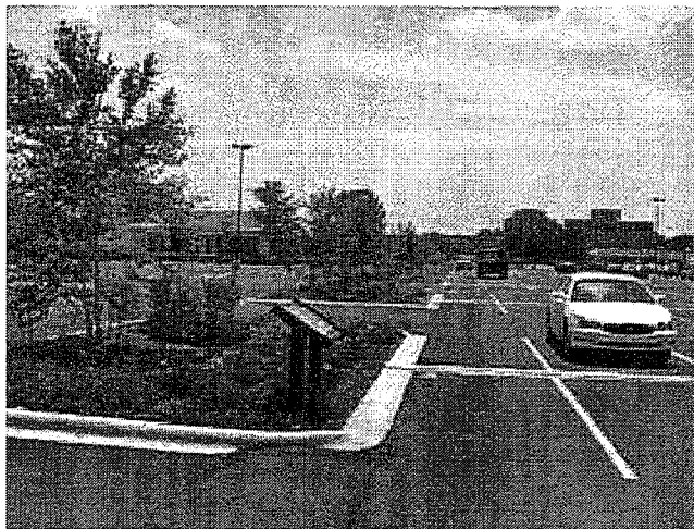
FIGURE 5-27 North Carolina Retrofit Bioretention SCMs. SOURCE: Traver.
