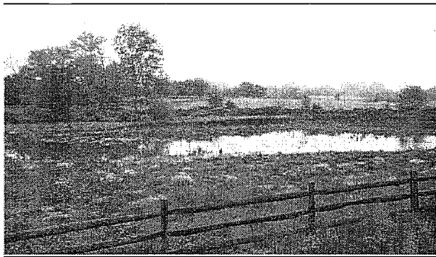
FIGURE 5-42 Wet pond. SOURCE: PaDEP (2006).
