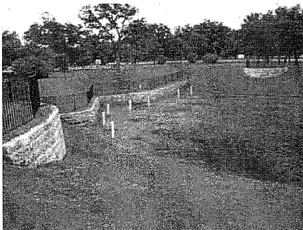
FIGURE 5-45 Austin sand filter. SOURCE: Robert Traver.
