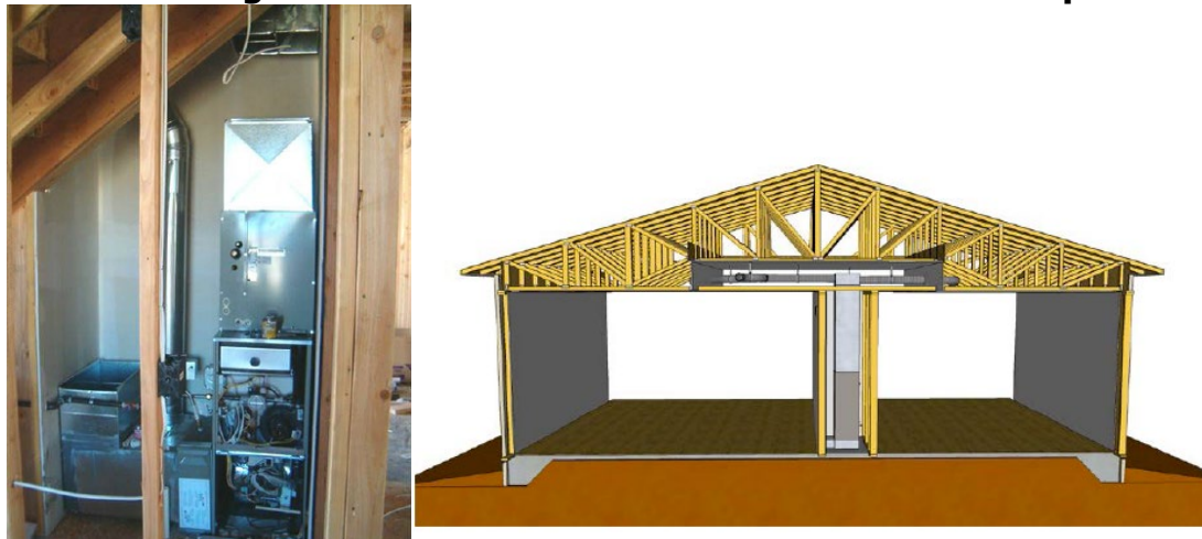
Figure 4-14: Mechanical Closet Placement Example
