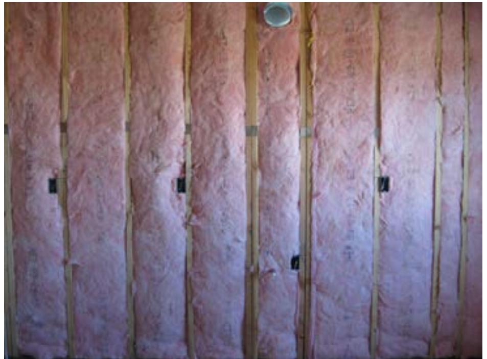
Wall Insulation – Third-party HERS verification of Quality Insulation Installation (QII) is now a prescriptive requirement for low-rise residential buildings. Source: California Energy Commission
