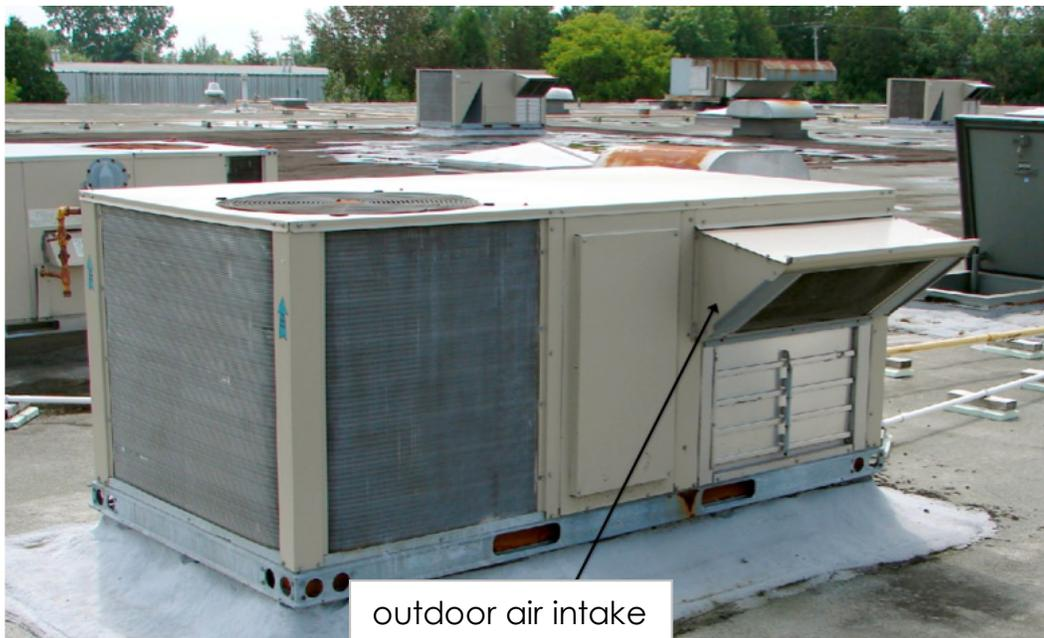
Figure 4. Outdoor air inlet for a typical rooftop HVAC system.
