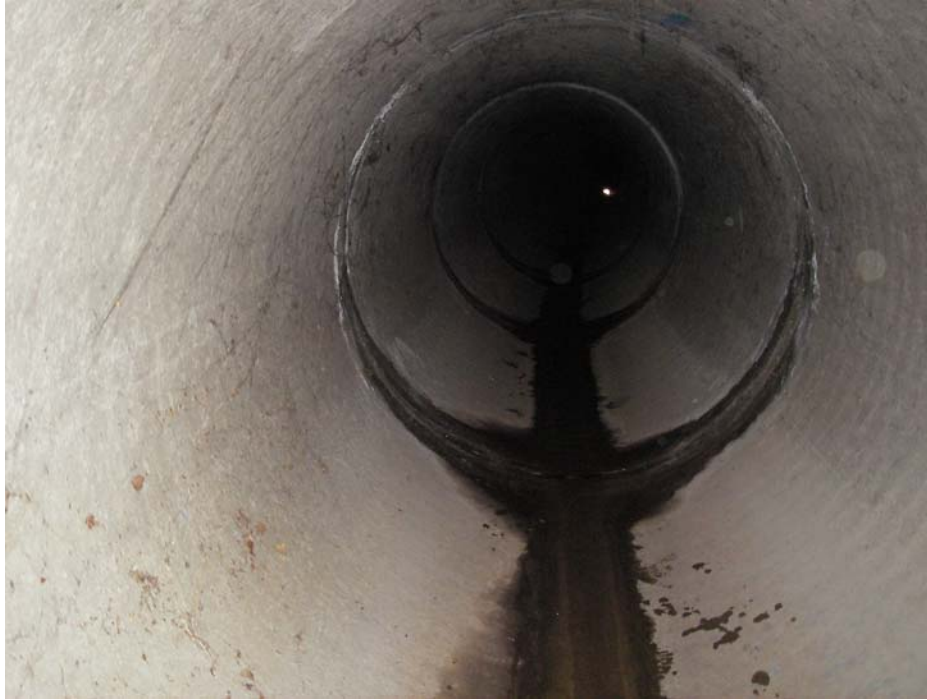
Figure 14. Evidence of groundwater seeping through conveyance pipes contributing to flows in Buena Vista Creek.
