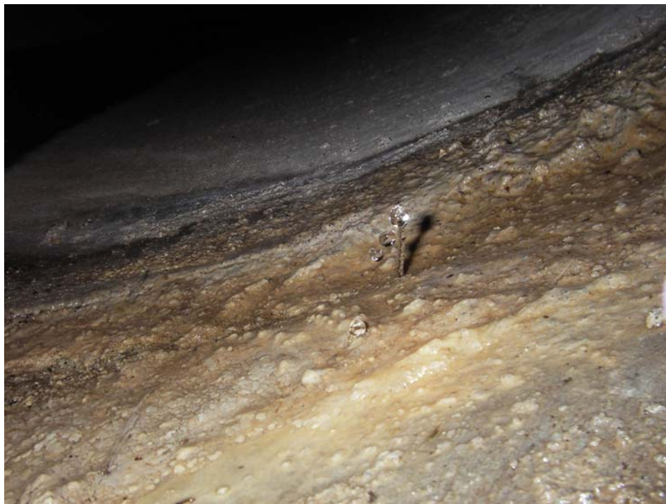
Figure 15. Groundwater with elevated nitrate concentrations seeping through cracks and seams in storm water conveyances in the Buena Vista Creek-HA.
