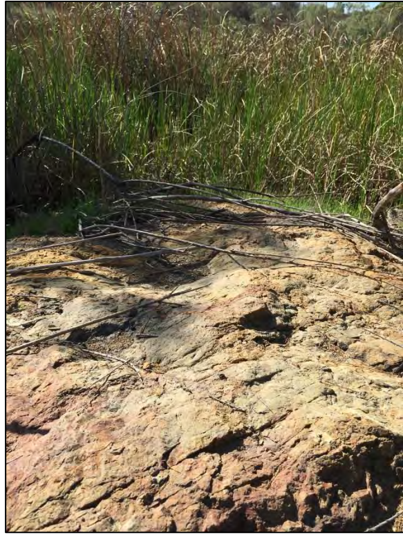
Figure 11: Cross Section 1 – Scoured to Bedrock
