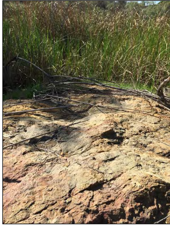
Figure 11: Cross Section 1 – Scoured to Bedrock
