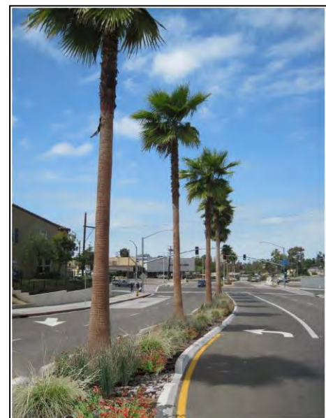
Bioretention swale on Logan Ave
