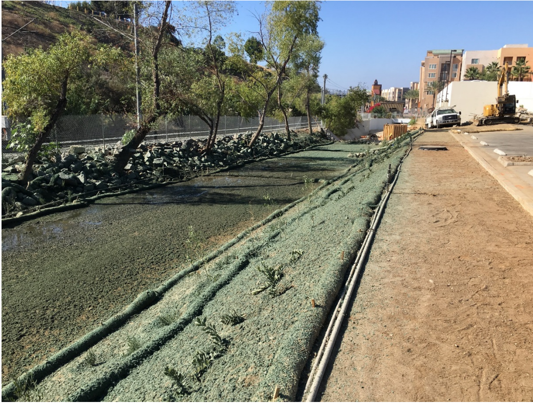
Figure 4-1. Alvarado Creek Restoration
