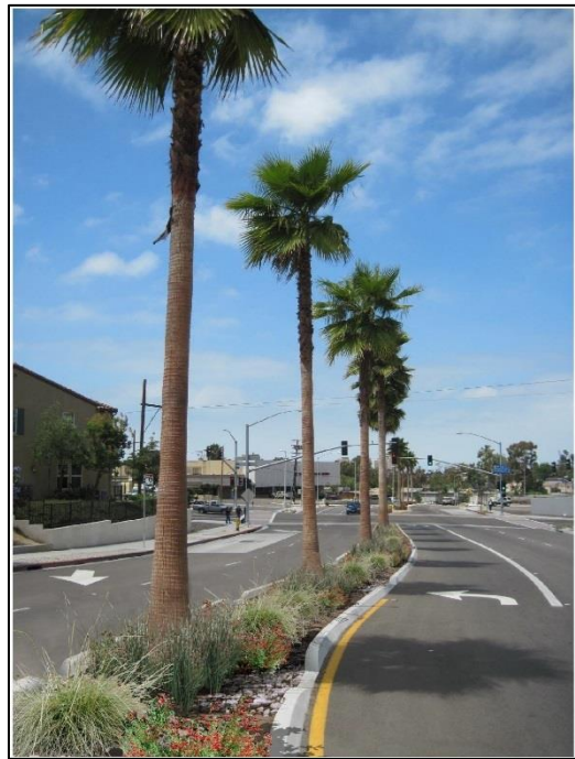
Figure 4-3 LID Incorporated into a Roadway Median
