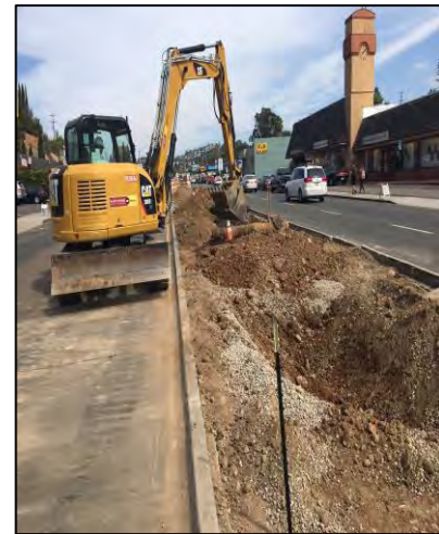
Replacing impervious areas with bioretention areas along University Avenue
