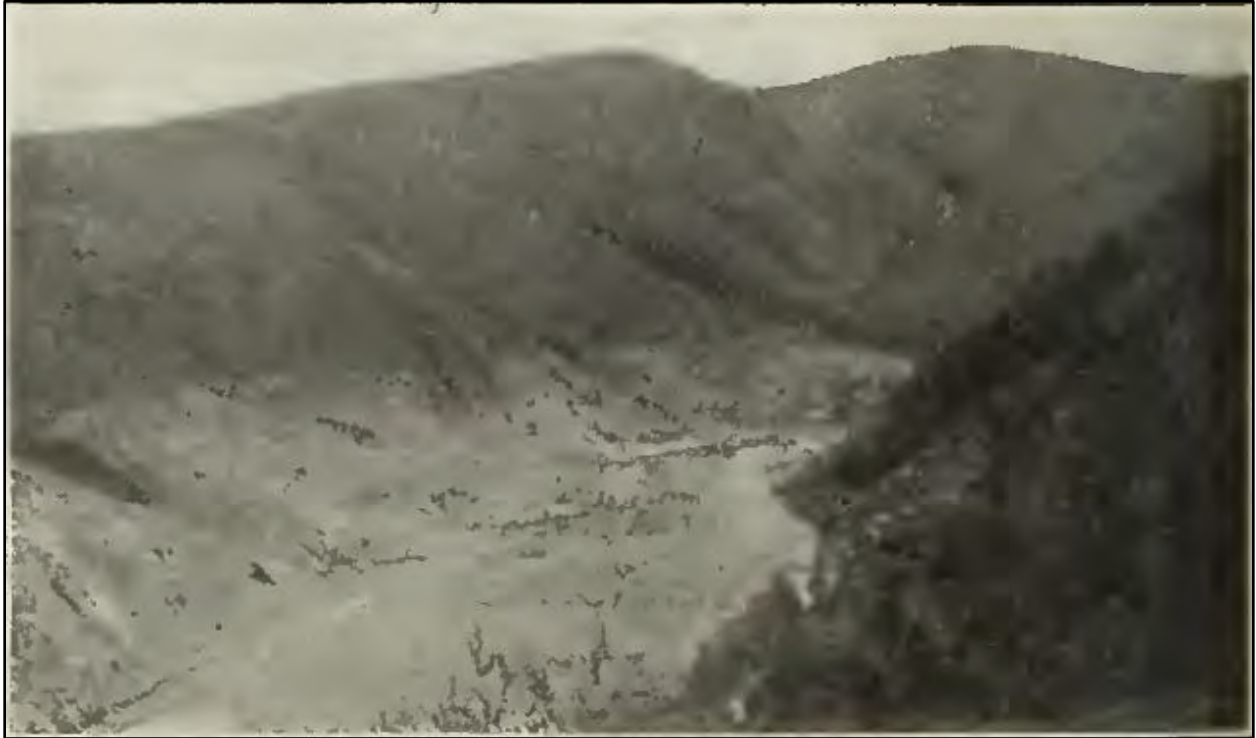
Figure 3: Canyon Immediately Below Dam, Showing Stripping Action of Water (Silent, 1916)
