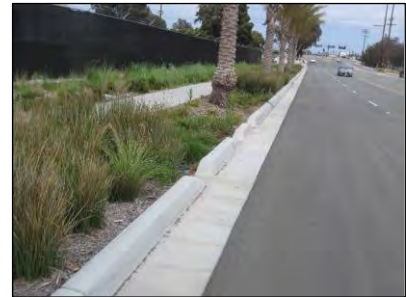
Bioretention facility at H Street Extension
