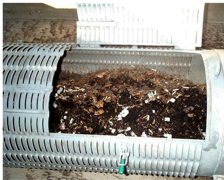
This Gross Solids Removal Device captures debris carried by water, which then flows back into the drainage system. The solid matter is then collected for disposal.
