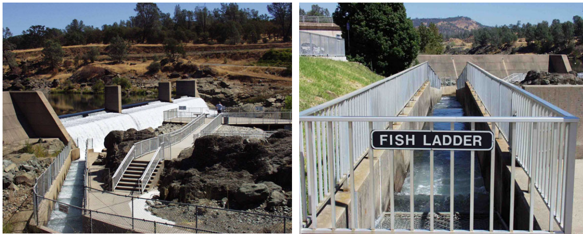
Figure 7.16 Fish Ladder at Feather River Hatchery, Oroville Dam, CA (Feather River, n.d.)
