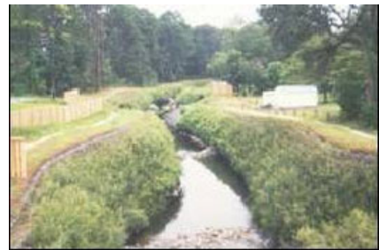
Figure 7.33 Established VRSS Structure (Sotir and Fischenich, 2003)
