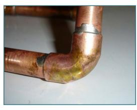
Copper pipes joined by lead solder.
