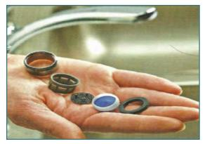
• Rinse the pieces with water and brush off the debris. For deposits that are difficult to remove, soak the parts in water for a few minutes and scrub with a toothbrush. Backwashing aerator components is also an effective cleaning method for many aerator types. Hold the removed aerator upside down under flowing water to backwash screens and mesh filters;
