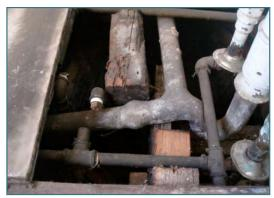
Example of lead pipes in a plumbing system.
