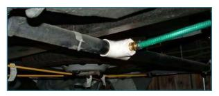
A garden hose creates a dangerous cross connection between potable and non-potable water.
