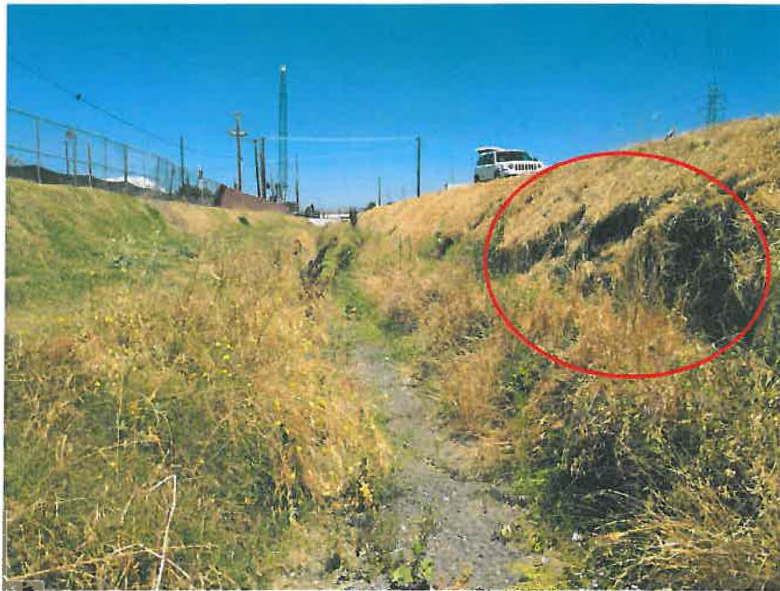
Figure 3A: Bank erosion upstream of Montague Expressway
