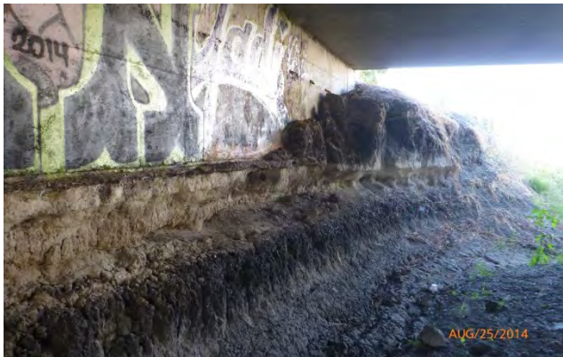
Top: Typical Reach 3 stretch. Bottom Left: Erosion under Yosemite Drive Bridge pier. Bottom Right: Looking downstream toward Yosemite Drive.
