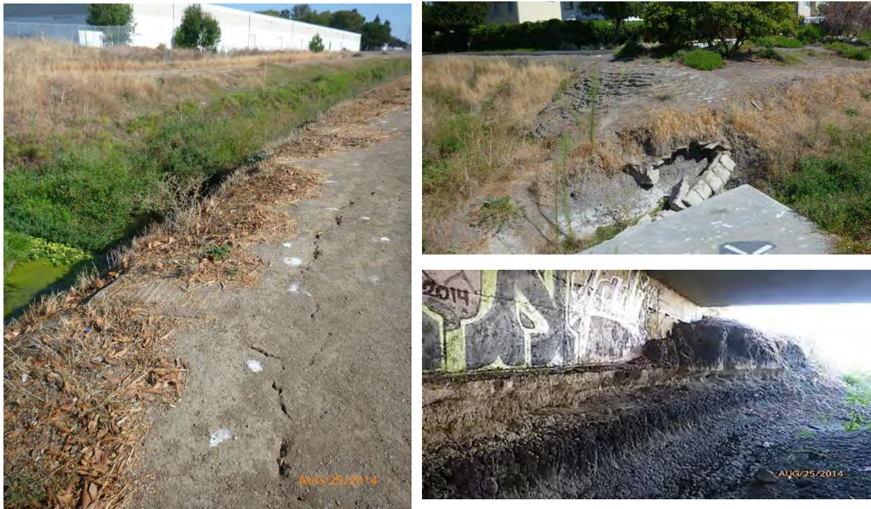
Left: Crack or fissures that indicate potential slumps. Note erosion control matting to left of crack. Top right: bank hardening that has become undermined by a lowering channel invert and high flows. Bottom right: Erosion beneath bridge piers.
