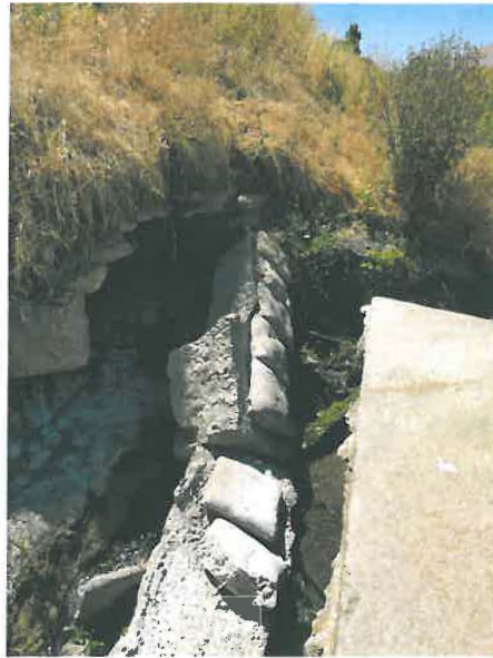
Figure 6A: Erosion upstream of Los Coches Street
