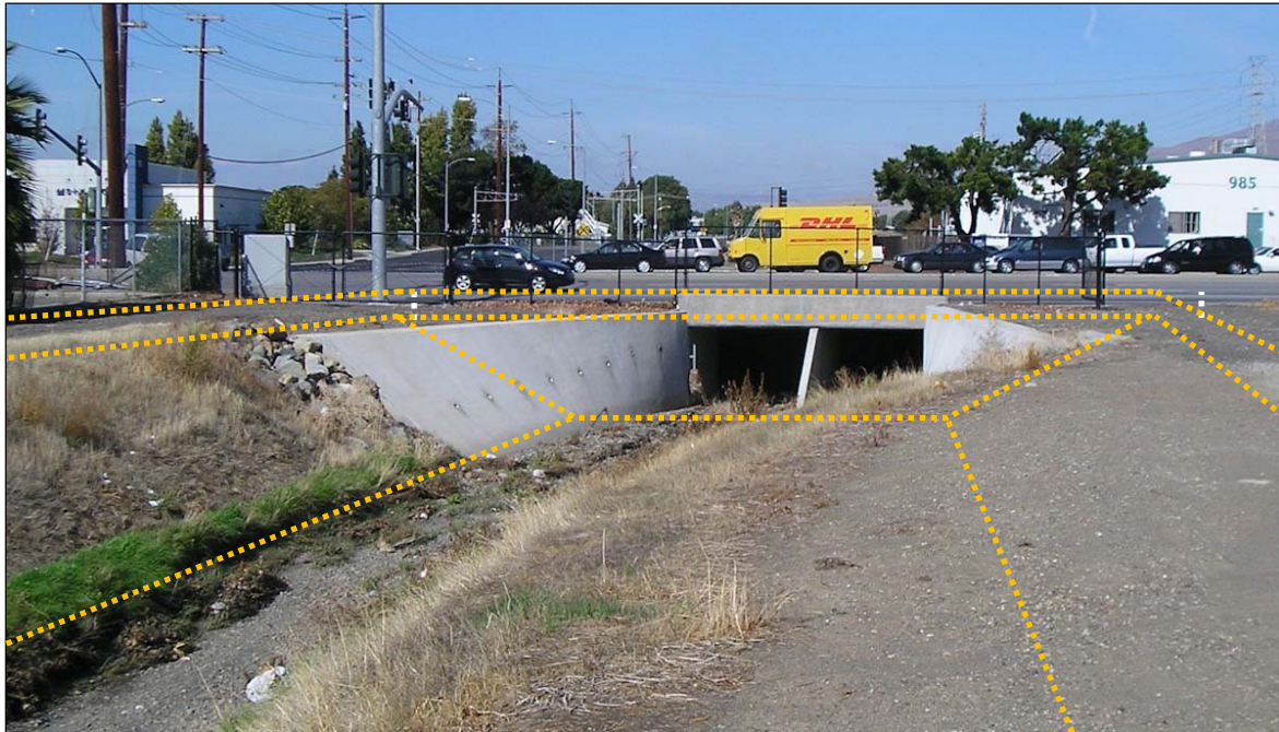
Figure 3-13 Schematic View of Montague Channel Excavation for Alternative 2B/d
