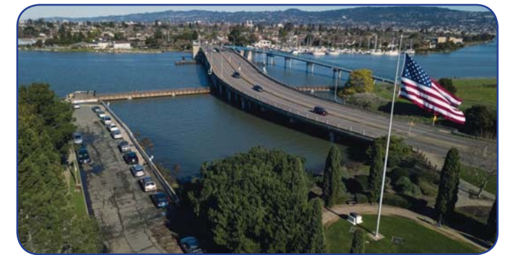
The City of Alameda's Clean Water Program maintains the storm drainage infrastructure which protects homes, property, and streets from flooding and protects the City's beaches and the Bay from trash and pollutants caused by urban runoff during rain events.
