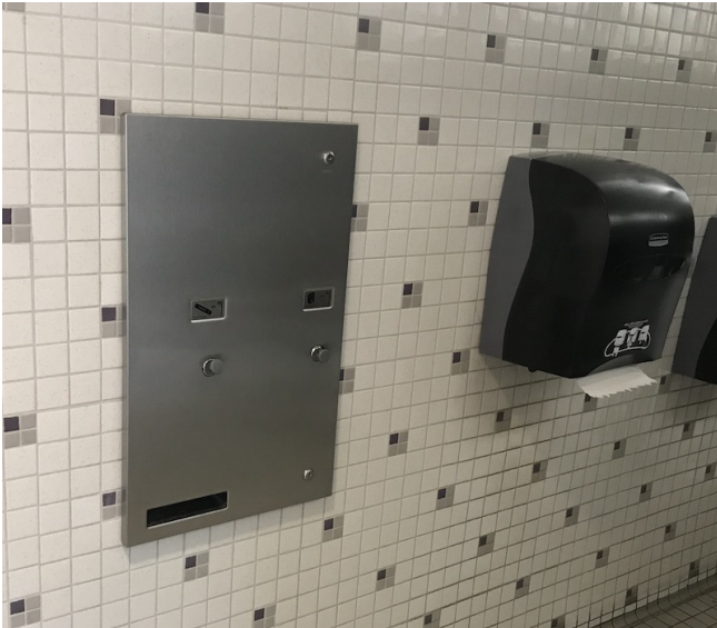
Several Berkeley High restrooms already have menstrual product dispensers. Photo: Natalie Orenstein
