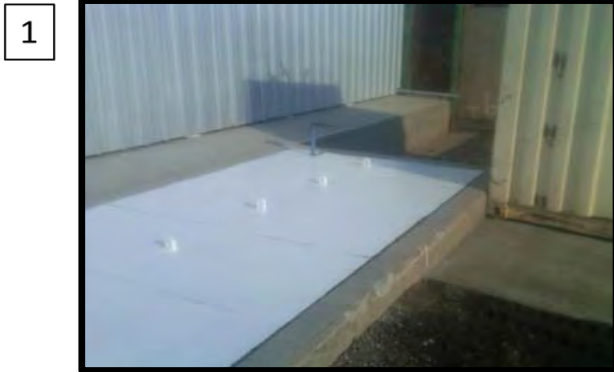
Coating steel to prevent rusting
