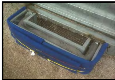
Adding filter cloth to structural filters
