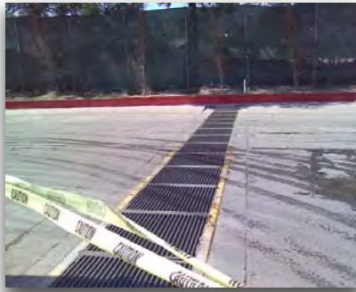
Gate capture devices for intercepting run-off
