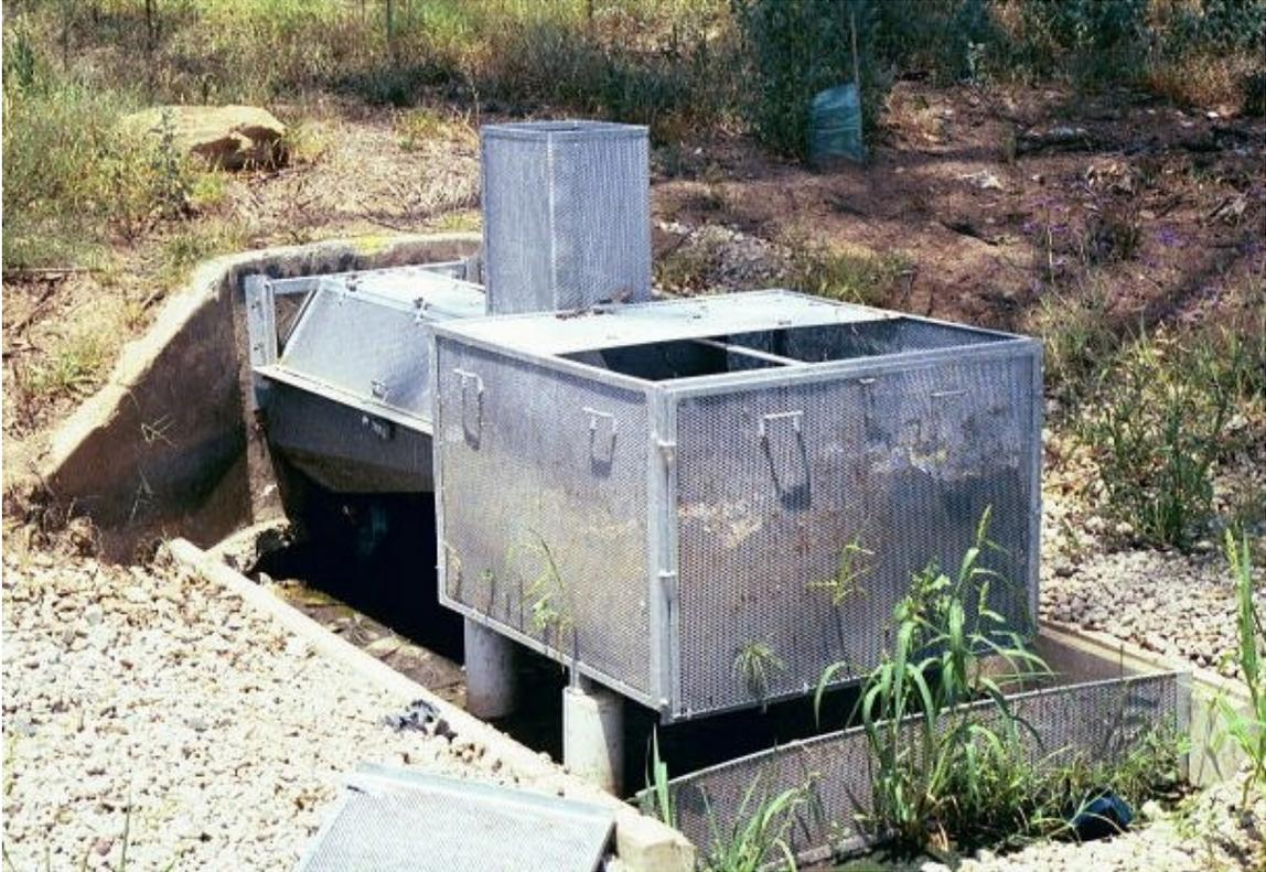
**Figure 3-4 Ski Jump Silt and Litter Trap®**
