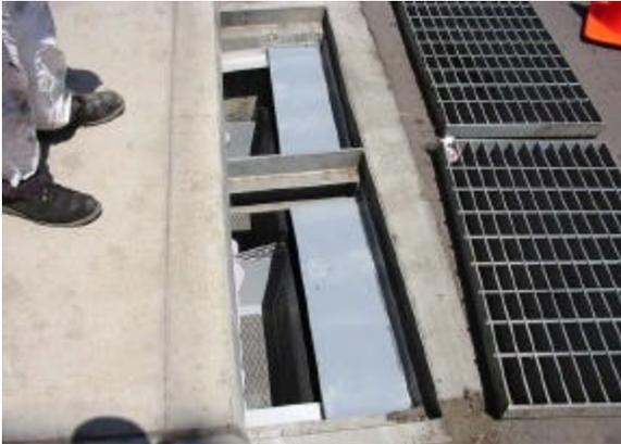
**Figure 3-15 BioClean™ Insert**
