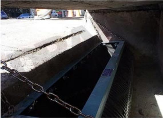
**Figure 3-13 DrainPac™ Insert**
