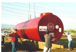
Underground storage tank
