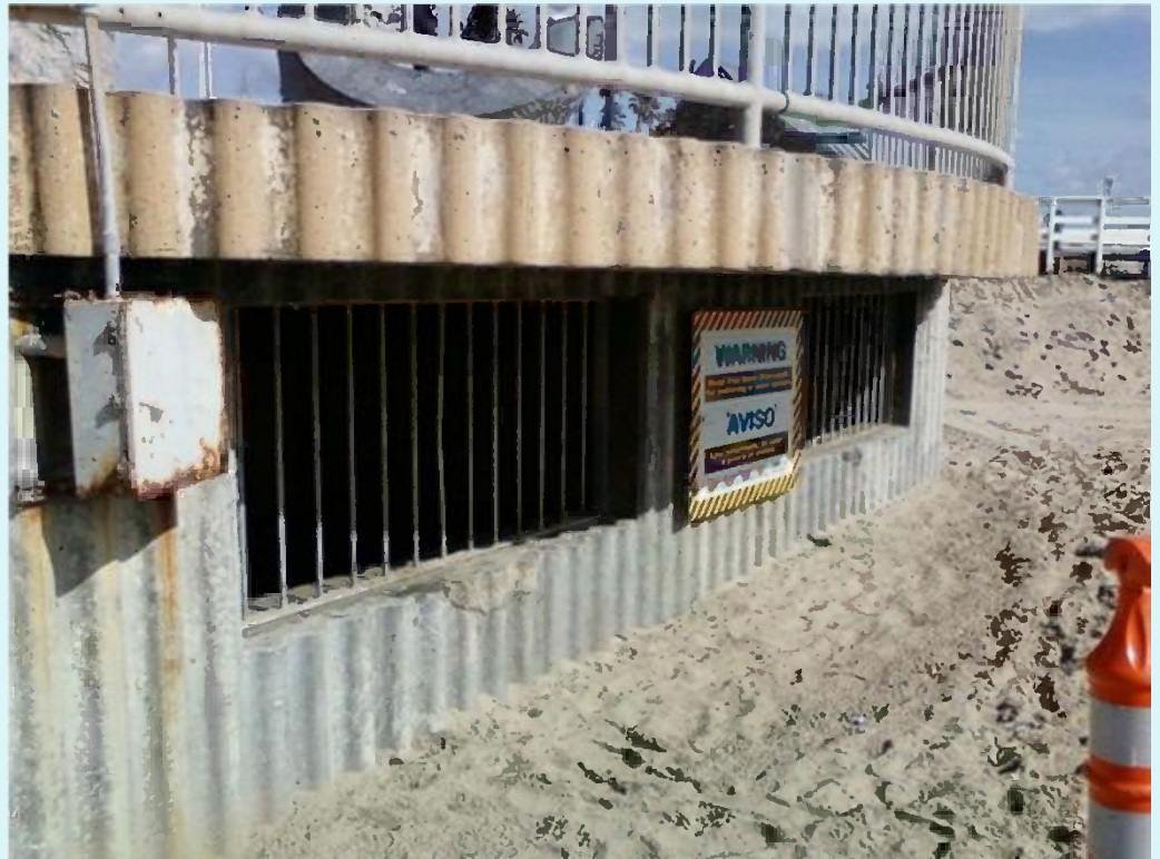
Neary Lagoon Beach Outlet Vault
